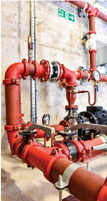
GRINNELL Mechanical Grooved HVAC System Installation
