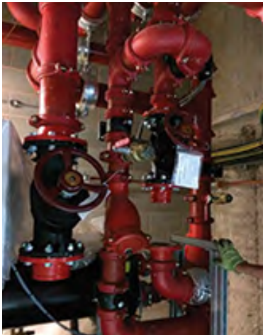
GRINNELL Mechanical Grooved HVAC System Installation
