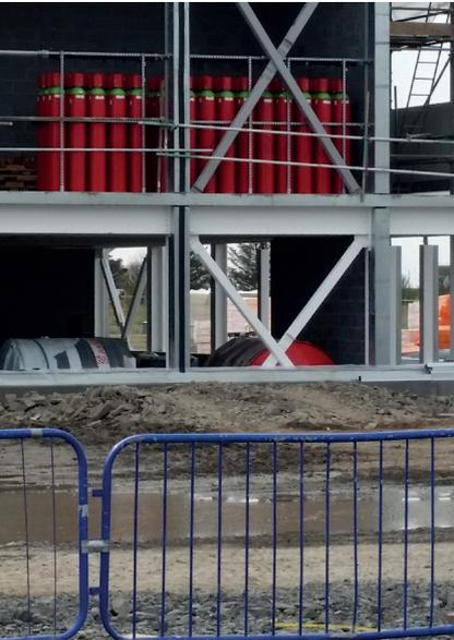
The iFLOW selector valves are calibrated to send the right amount of gas to wherever the fire is burning and it is the design of the delivery pipework that sets the Nucleus installation apart. More traditional designs would site all eight selector valves alongside the remotely positioned gas storage cylinders, requiring eight pipe runs to take the gas to each room. APL has positioned individual valves outside each room, all feeding off just one run of pipework.
